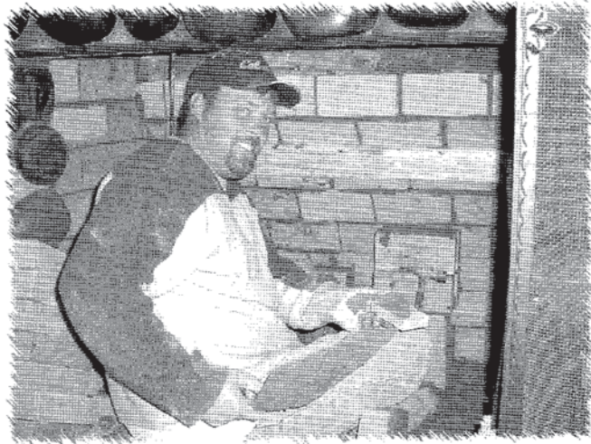
Jared "Hoss" Nielson rebuilding Sunnyside Resort's massive firebox.
